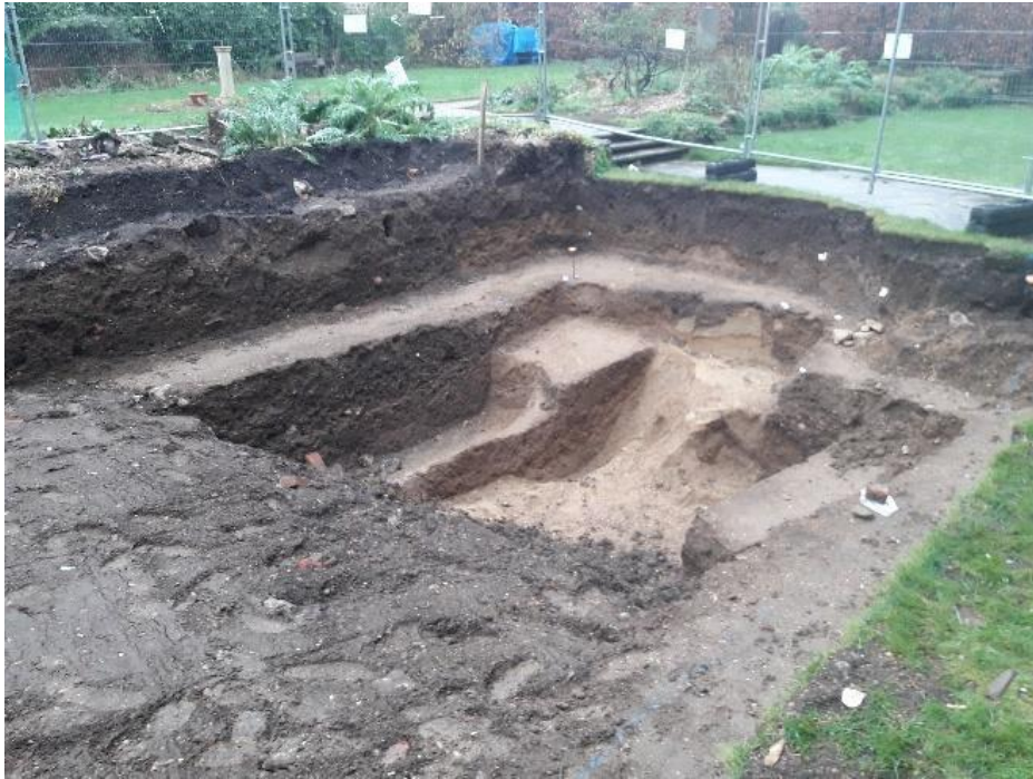
Image 2: Excavation for storm water tank
