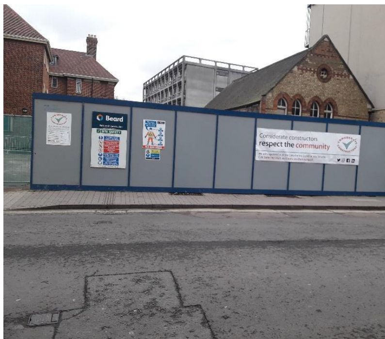
Image 1: Hoarding to be moved to road edge
